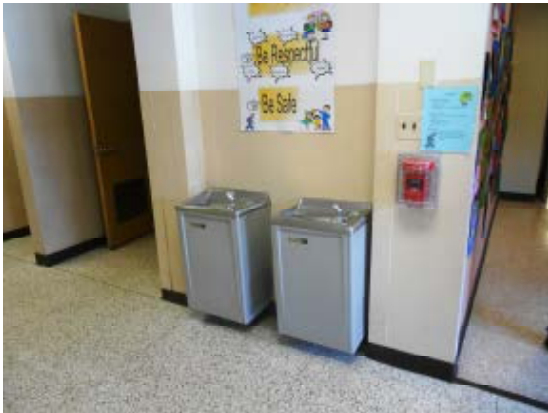
Non ADA compliant water coolers
